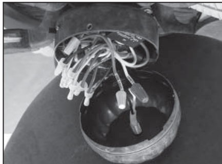
5. Connect white-to-white and blue-to-black wires with wire nuts.
