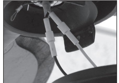
3. Connect white-to-white and blue-to-black wires.
